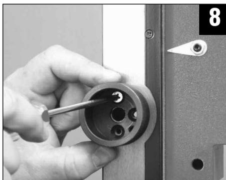
8 Install spring support to left side of column with 3 screws.
