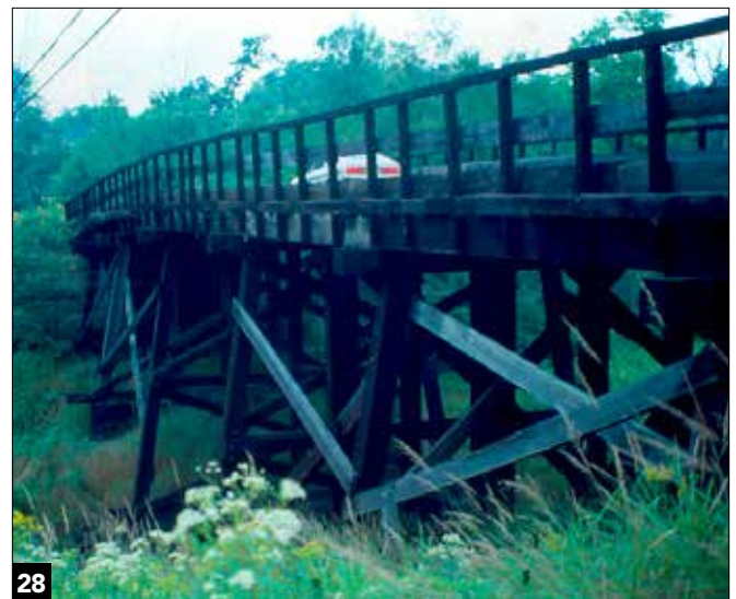
28 Road overpasses built from wood can still be found in rural areas on secondary roads. This would be another way to satisfy the trestle-building bug. CJ Riley
