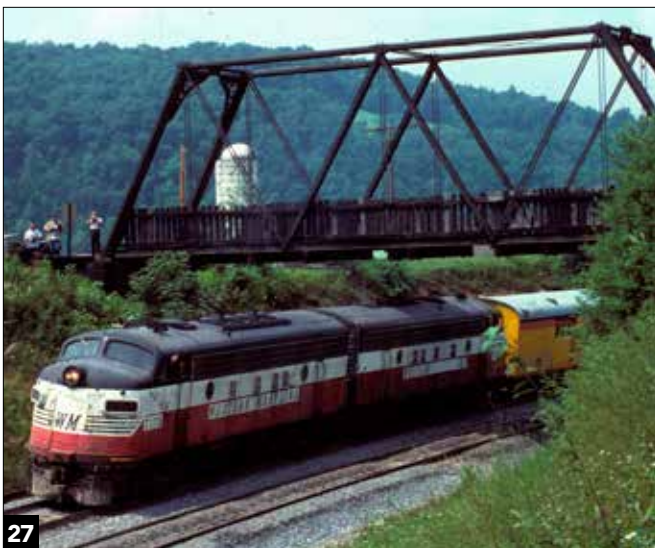
27 Railroads also go under bridges, frequently those of roads. This is a very old cast iron pin-connected truss bridge near Sand Patch Pa. CJ Riley
